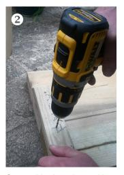
Start with the short sides. Lay the battens in place butting them up to the sides of the planks. Hold the battens securely and drill pilot holes.
