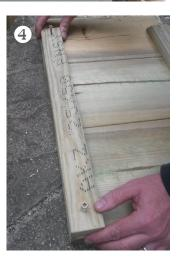
SCREW TOGETHER Line up the pilot holes and fix in place with timber screws. Repeat to build the other short side.
