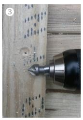
If possible, recess the screw heads to prevent the screws catching on the liner.
