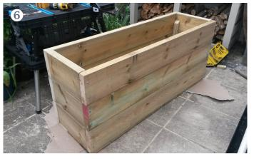
**ADD THE BASE** Turn your planter over and fix decking planks to form the base. Drill a hole in the side or end of your planter using a flat head bit or hole-saw - this hole wil take the plastic drainage pipe so position it accordingly. Drill some drainage holes in the base to revent rot.
